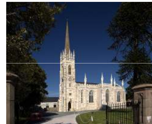
St Mark's Parish Church, Newtownards
